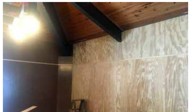
New plywood is installed.
